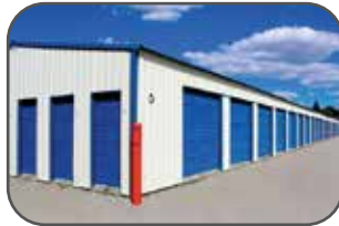
Remote storage units
